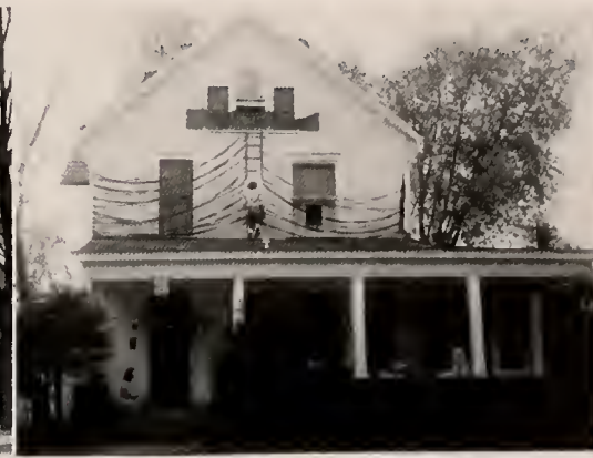
College Avenue House
